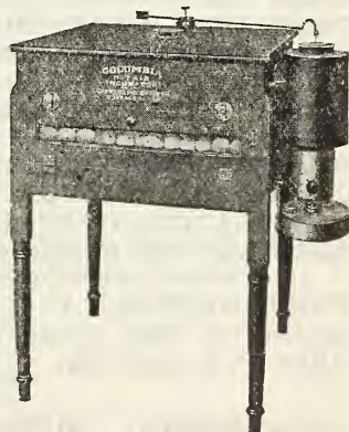
Small size Columbia incubator. Capacity, 140 eggs.
